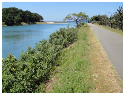
護岸のハマボウの植栽
